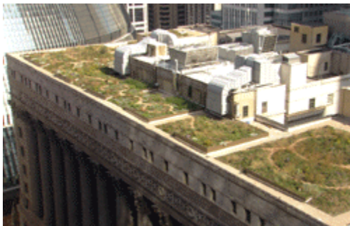
Figure III-5. Roof of Chicago City Hall
